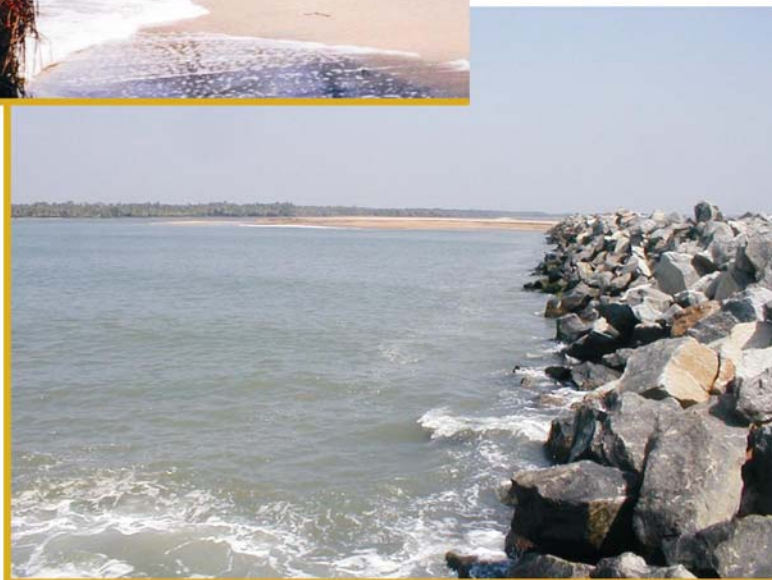
Figure 5.9 Coastal erosion in different parts of Ponnani
