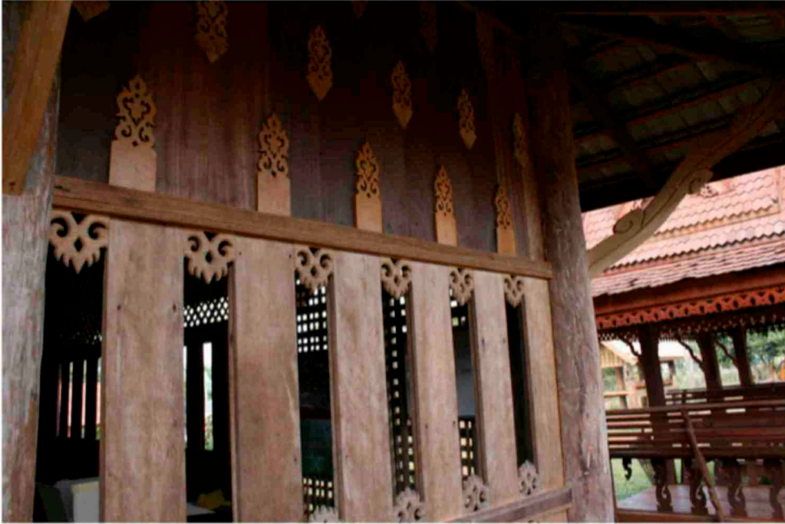
Fig. 74. Wooden decoration and paneled walls, sala for teaching of dhamma , Wat Pa'O Ram Yen.
