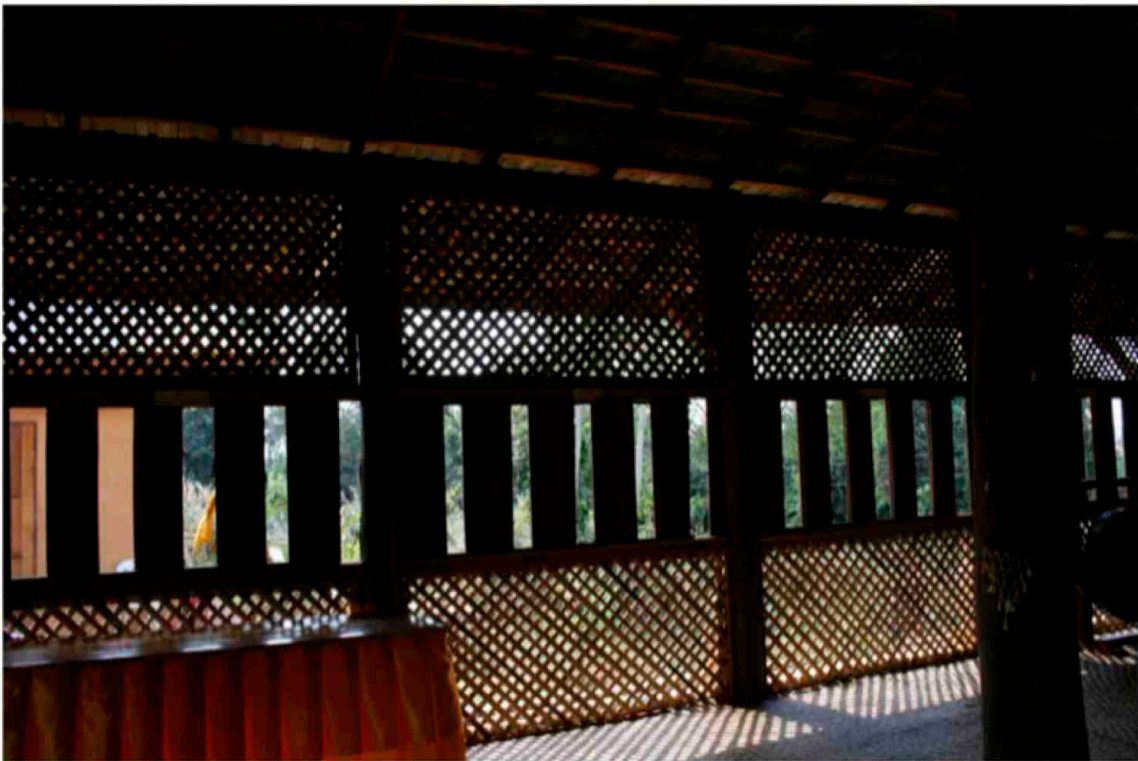
Fig. 75. Semi-opened wall, sala for the teaching of dhamma , Wat Pa'O ram Yen.
