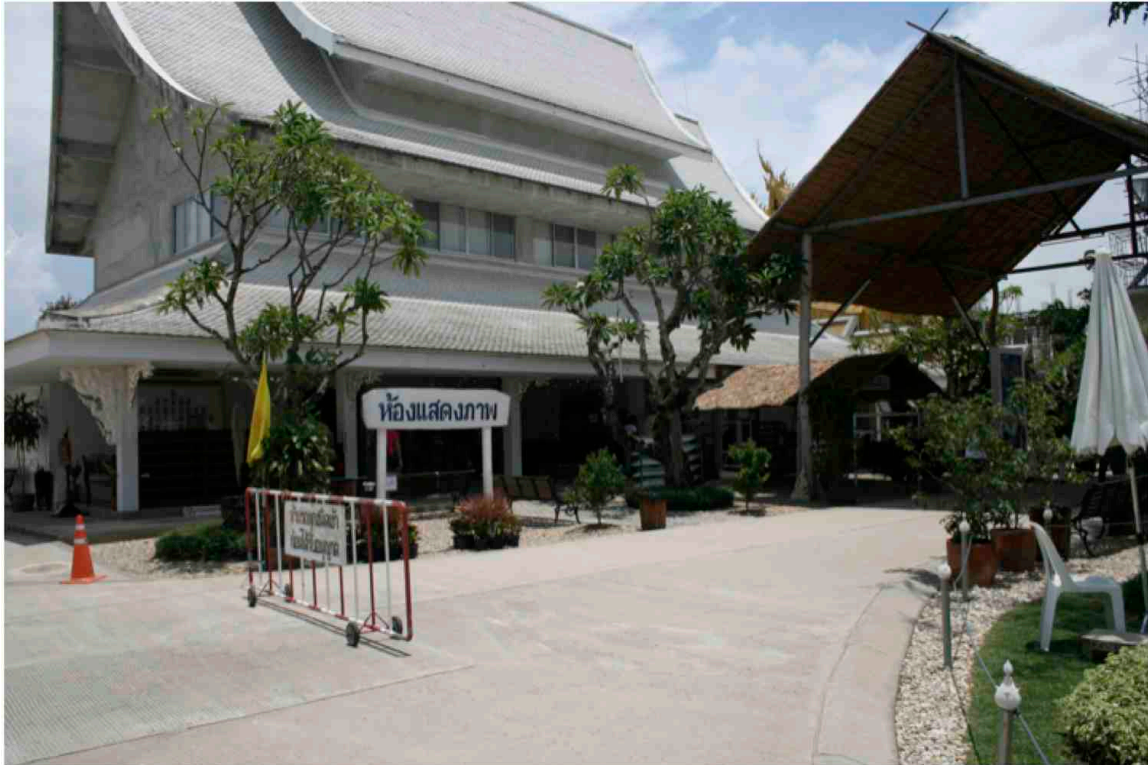
Fig. 35. Gallery, South-East entrance, Kharawat, Wat Rong Khun
