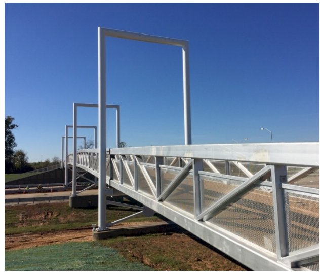
(b) Arthur Ray Teague Parkway Pedestrian Bridge Bossier City, LA, United States
