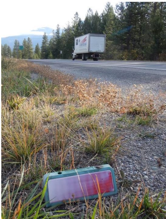
Figure 4.36 Decommissioned wildlife reflector installation
