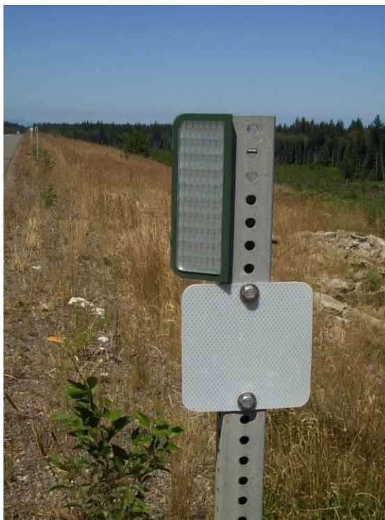
Figure 4.35 Wildlife reflector installed by a highway
