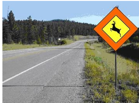
Figure 5.14 “Very High” Hazard
