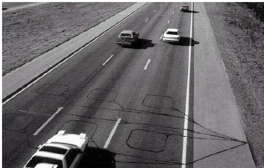
Figure 6.5 Inductive loops Source: US Federal Highway Administration
