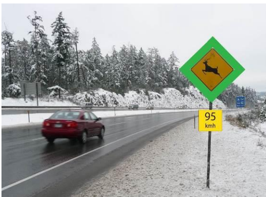
Augmented deer crossing sign at a low hazard period with advisory speed tab
