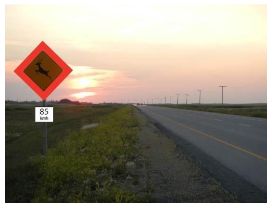
Augmented deer crossing sign at an extreme hazard period with regulatory speed tab
