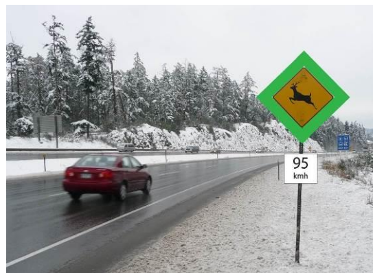
Augmented deer crossing sign at a low hazard period with regulatory speed tab
