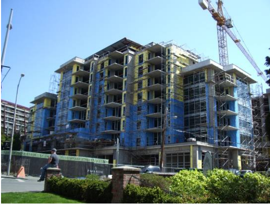
Construction on Humboldt Street, viewed from the St. Ann's Property
