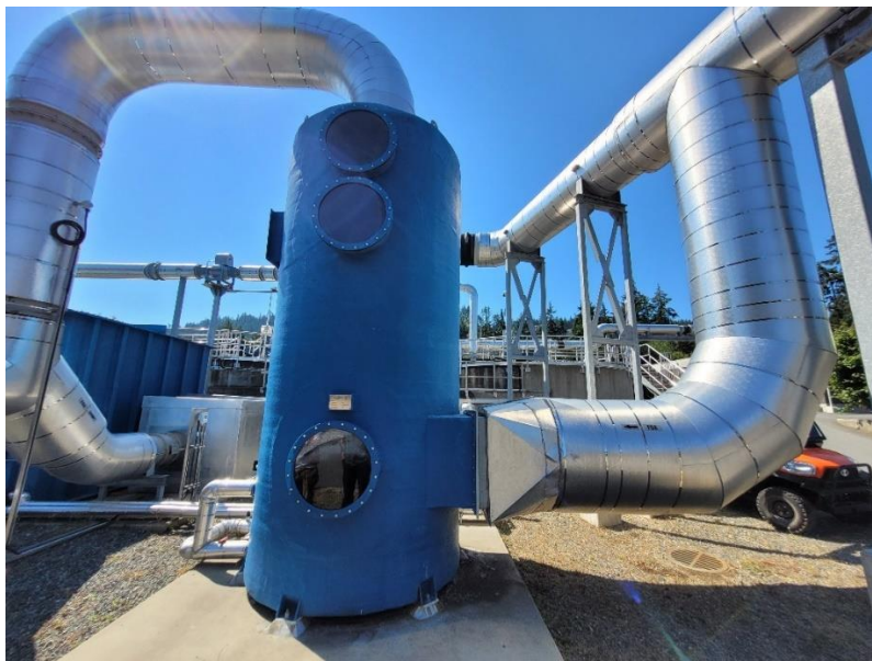
Figure 28 Photo of Rain tower, which adds humidity to the airstream before it enters the Bioreactor odour control, Exhaust of Rain tower to the left is sample point 8.
