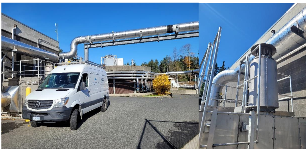
Figure 19: (Left) Photo of Mobile Mass Spec Lab on-site WWTP2 at sample locations 2 & 3, Modular activated carbon scrubber 1 to left of the MMSL. (Right) Photo of exhaust stack from Modular scrubber, sample point 3.
