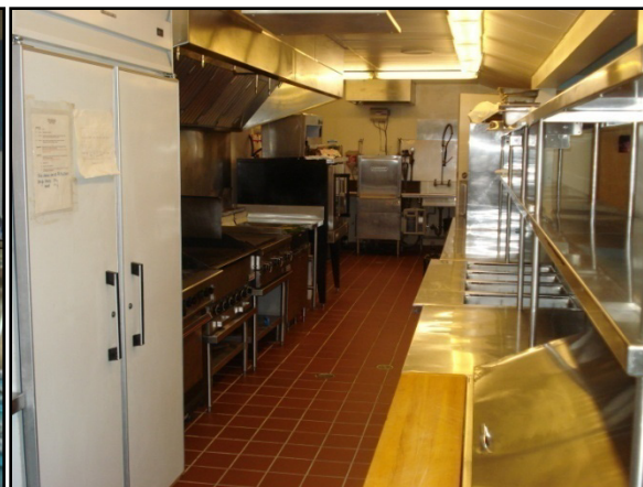
Gulf Islands Secondary, Cafeteria Kitchen
