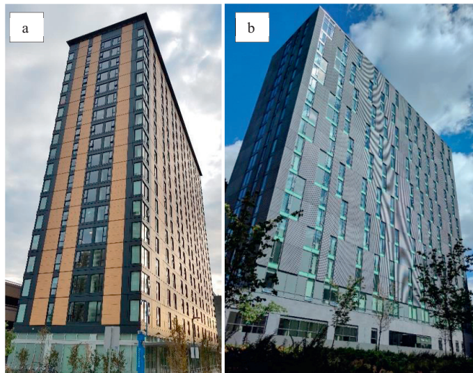
Fig. 1 Studied student residential tower at UBC (a) Brock Commons Tallwood House: Mass-timber hybrid structure (b) Ponderosa Commons Cedar House: concrete structure (photos by: Zahra Teshnizi)
