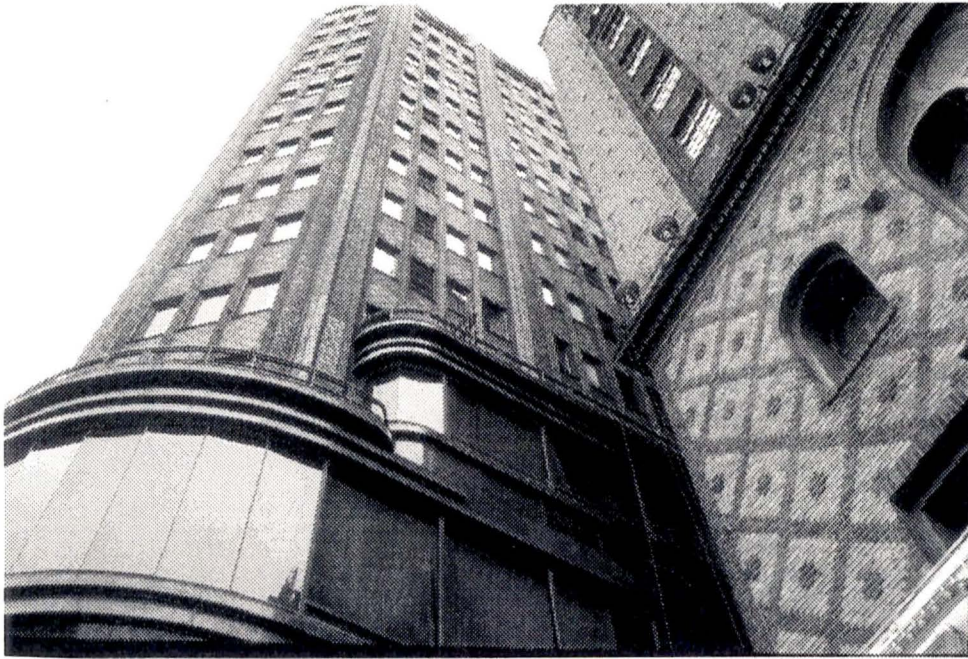
Fig. 27. Park Hotel. Detail of corner, next to Y.M.C.A. Scanned photograph. Source: Dr. Jeffrey Cody, April 1996.
