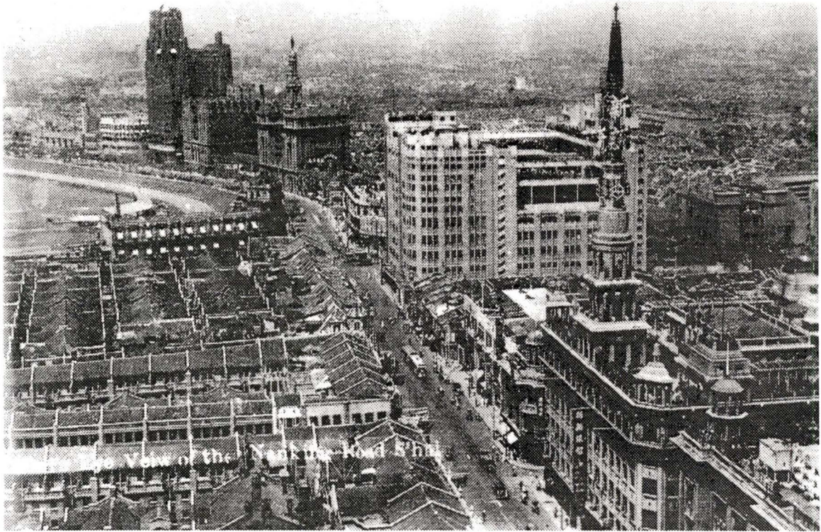
Fig. 37. Park Hotel and surrounds. View west from the Bund. Scanned image. Source: Deng and Zhou, Shanghai Survey, 1840s-1940s , p. 67.
