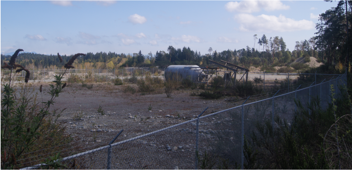
Figure 7.6: Decommissioned mine site, Nanaimo River Road
