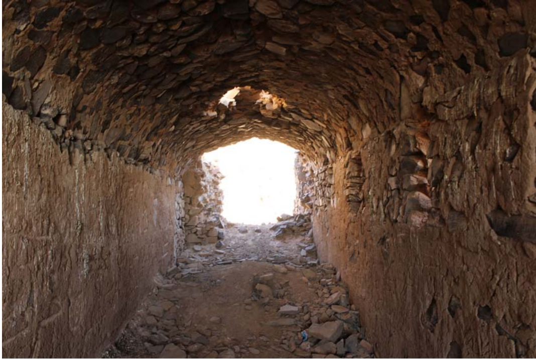
Figure 5-23: Stone pointed barrel-vault without a course of brick at the springing line, Kuh-Qal'ih of Tun. Credit: Author.
