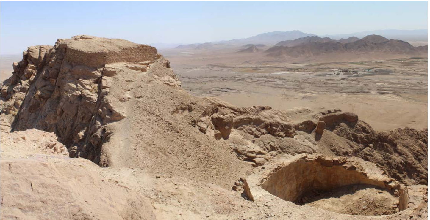
Figure 4-69: Qal'ih-Dukhtar of Shurab, building CB viewed from the top of the building CA. The cistern in the southeast corner of CA is seen on bottom right. Credit: Author.
