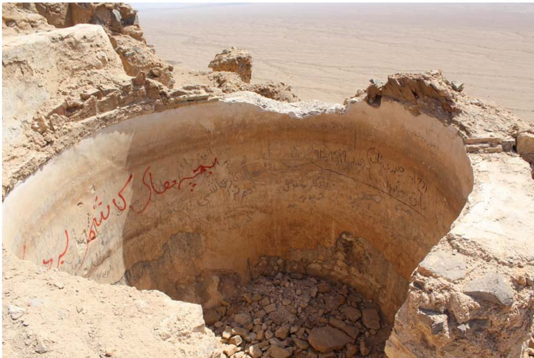
Figure 5-26: A circular pit (about 4 m in diameter and at least 3.5 m in depth) in the highest section of Qal'eh-Dukhtar of Raqqih. The pit was covered by a brick dome built of girdchīn technique as suggested by the remaining two courses of bricks.
