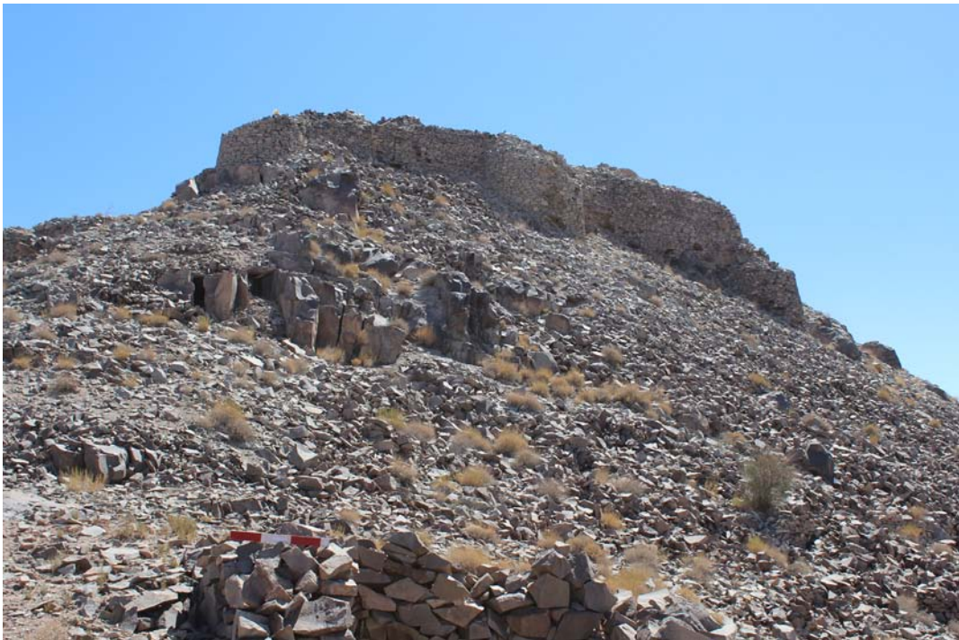
Figure 4-52: Qal'ih-Rustam of Khusf, section C's western curtain wall, viewed from section B. Credit: Author.
