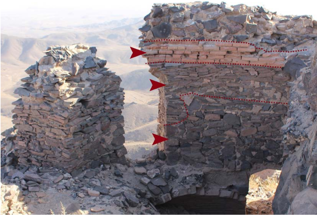
Figure 5-27: Remains of a wall from an interior structure with mixed use of material in the north of the highest part of Kuh-Qal'ih of Tun.
