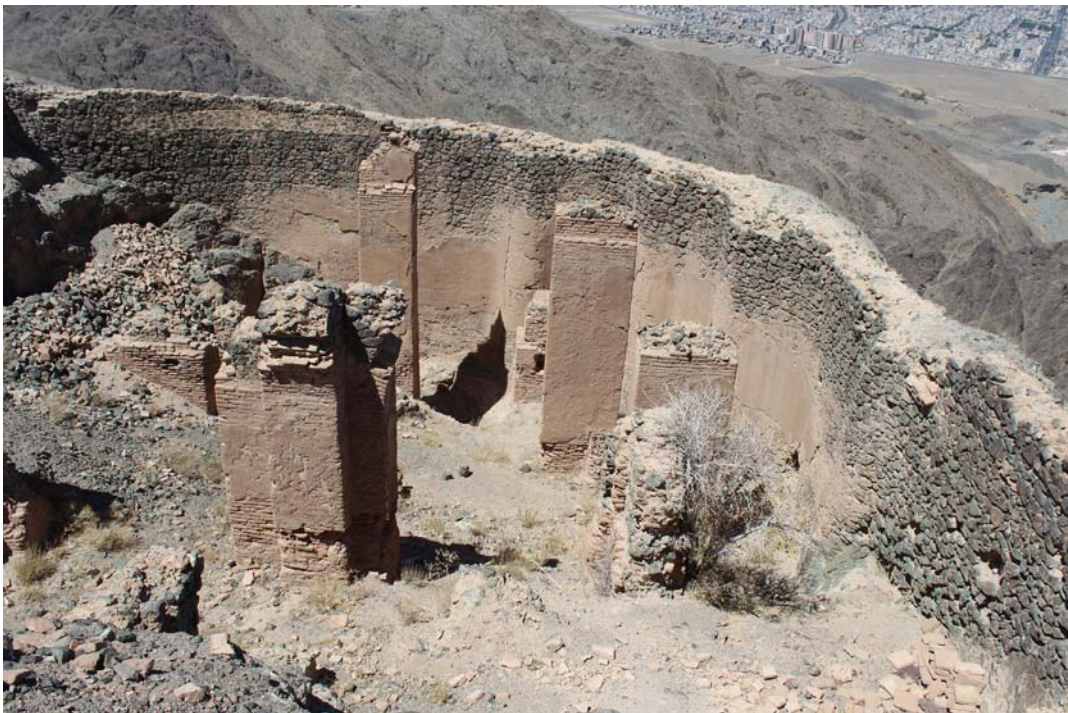
Figure 4-42: Castle of Darrih, Hawz-i Ghulam-Kush in section A, viewed from the southeast. Credit: Author.
