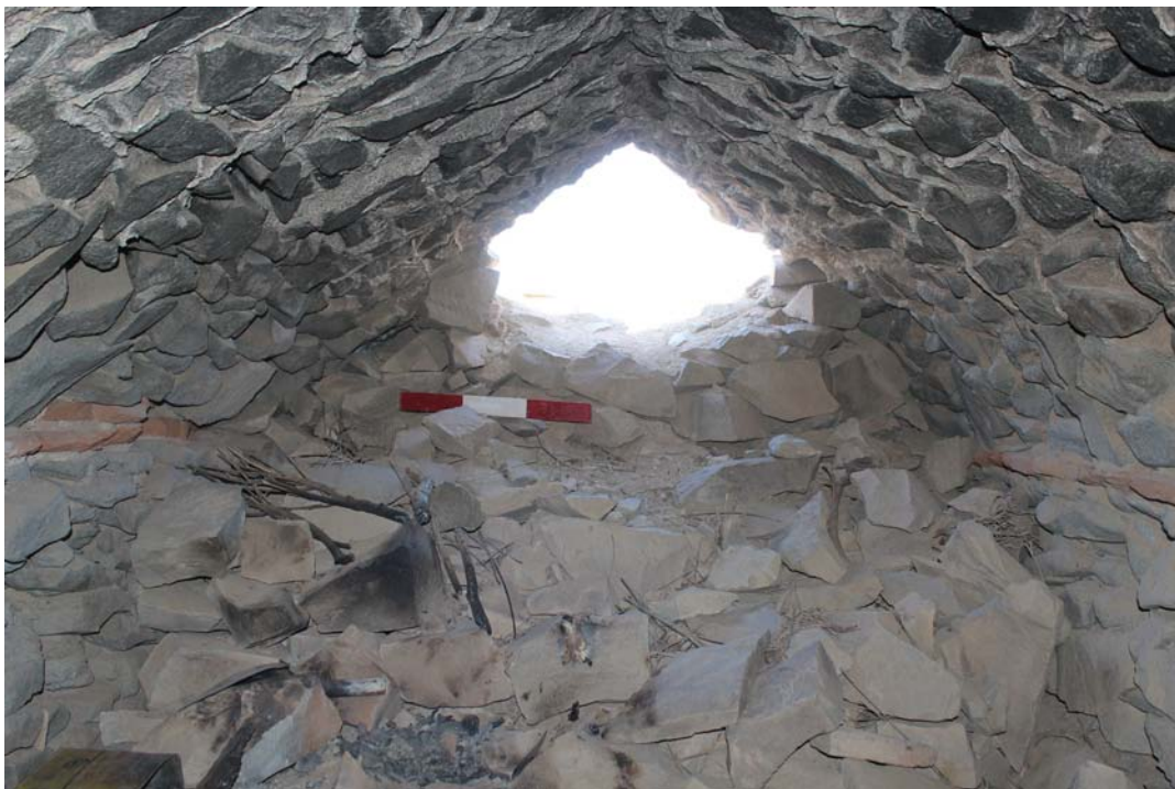
Figure 5-22: Stone pointed barrel-vault built on a course of brick at the springing line, Qal'ih-Rustam of Khusf. Credit: Author.
