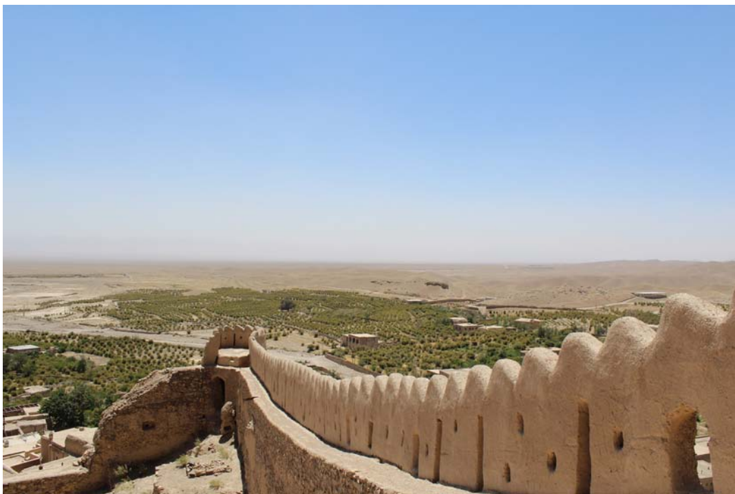
Figure 5-28: Furg castle, the remains of the mud-brick battlements and the narrow walkway (allure or wall-walk). Credit: Author.
