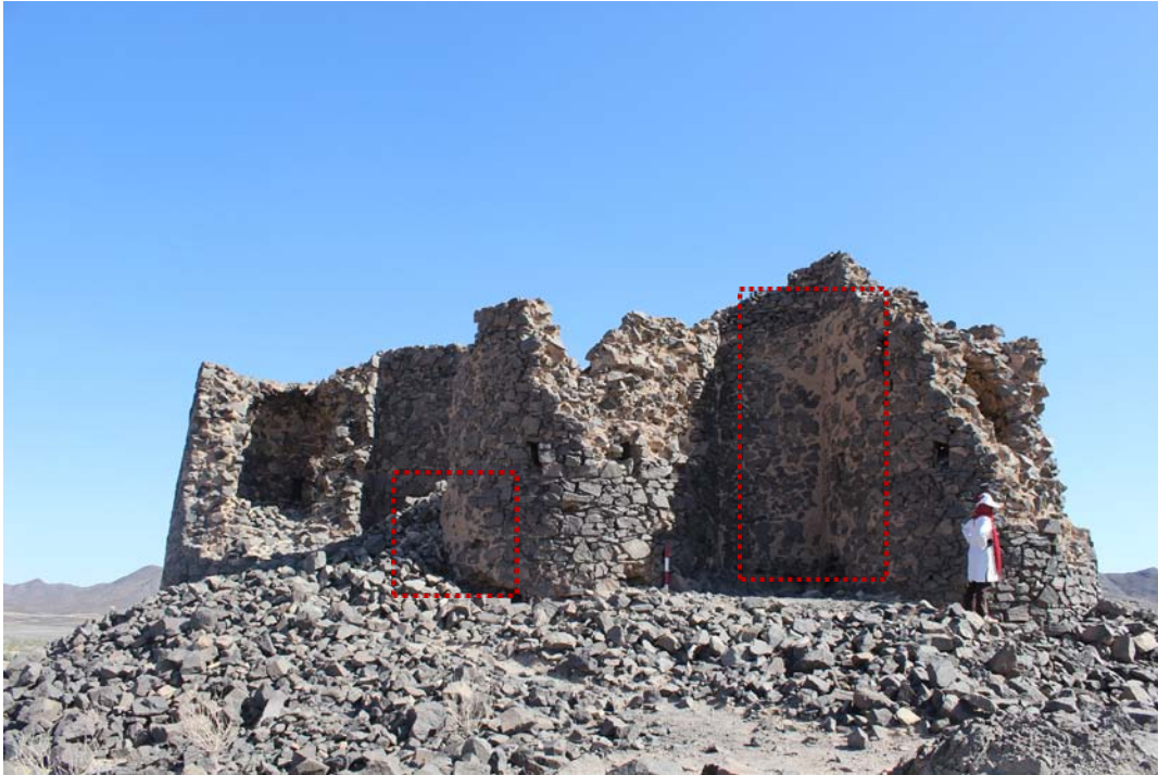
Figure 4-62: Northern flank of Qal'ih Zari. Note the traces of plaster remained on the walls. Credit: Author.
