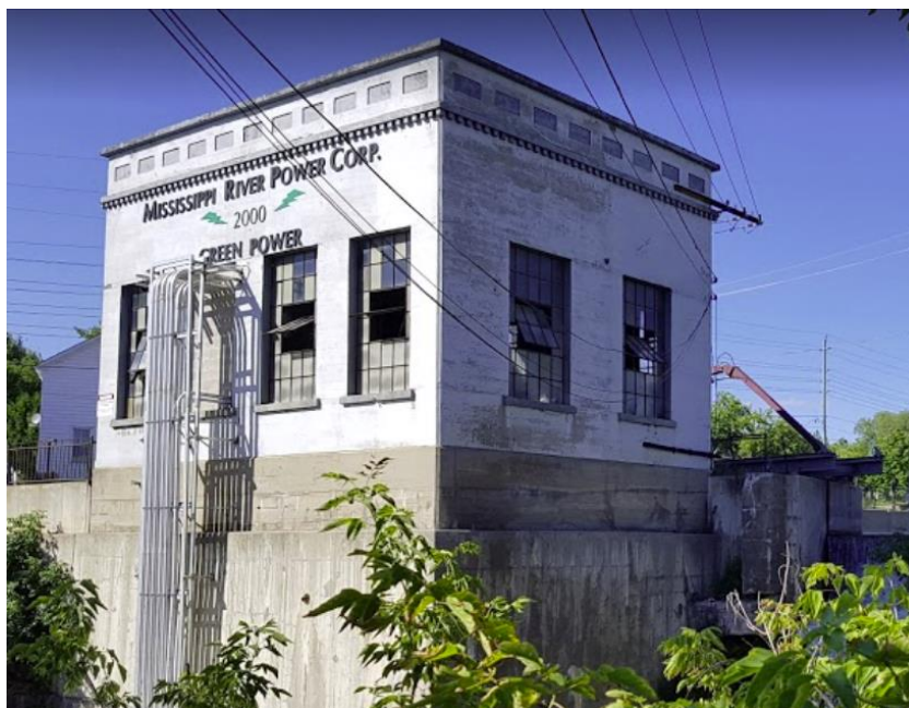
Figure 14: Almonte Power Plant, Almonte, ON. View from the outside (copyright: Google Maps/Google Earth).
