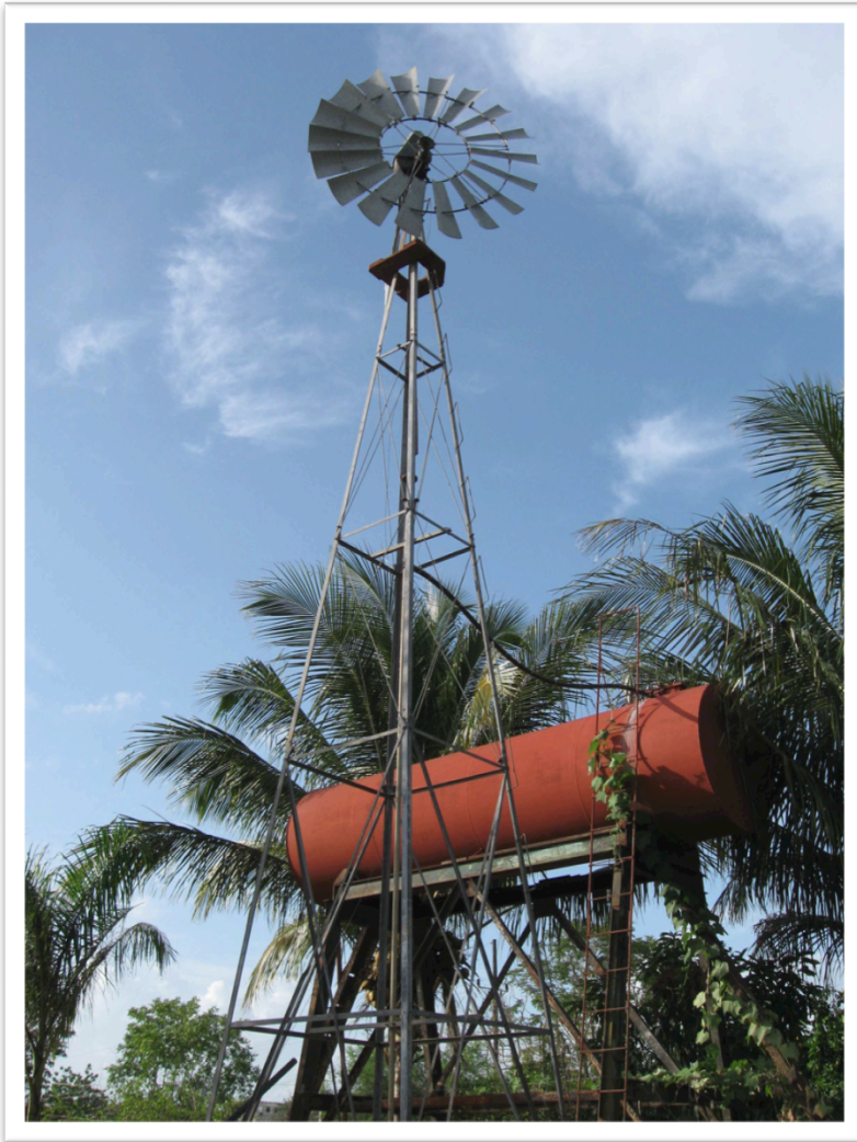
Photo 10: PDP photo taken by Participant 4 of things that support her in farming: Windmill- generates power for their electrical needs and decreases dependence on the electrical grid
