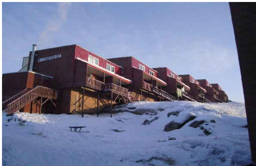
Figure 3.24 Housing in Lower Iqaluit, designed to follow the contours of the land.
