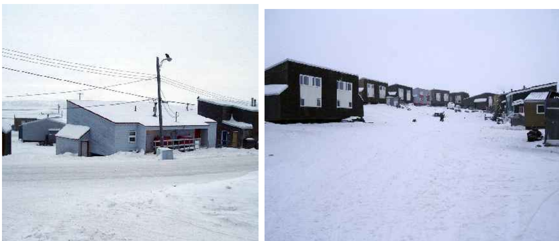
Figure 1.11 Example of houses with passive solar design. Large windows face to the south, and south-facing rooms have high ceilings. North faces have small windows and lower ceilings. The development pictured here is in Lower Iqaluit.
