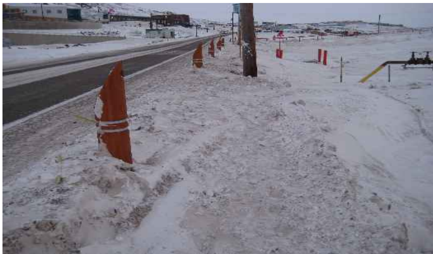
Figure 1.8 Wooden barriers on the Ring Road to define vehicle and pedestrian space.
