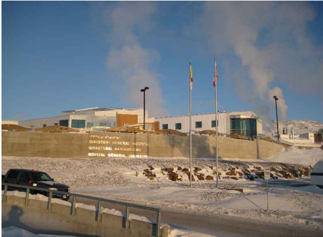
Figure 3.5 New building of Qikiqtani General Hospital, viewed from the Ring Road.
