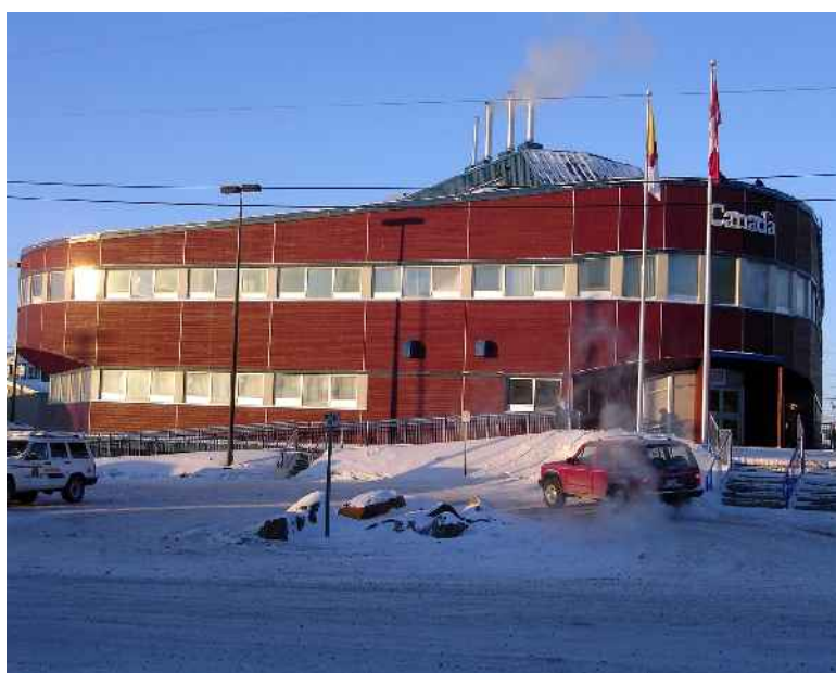
Figure 1.6 Government of Canada building.
