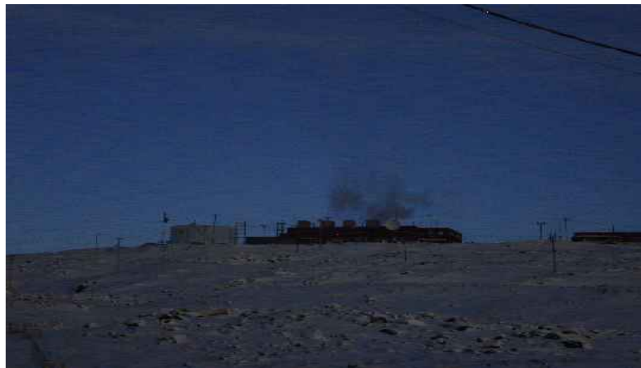
Figure 3.18 Power Station, on the ridge behind the Hospital and adjacent to the Plateau.
