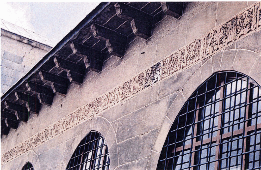
Figure 3. Diyarbakir Ulu Cami main prayer hall façade
