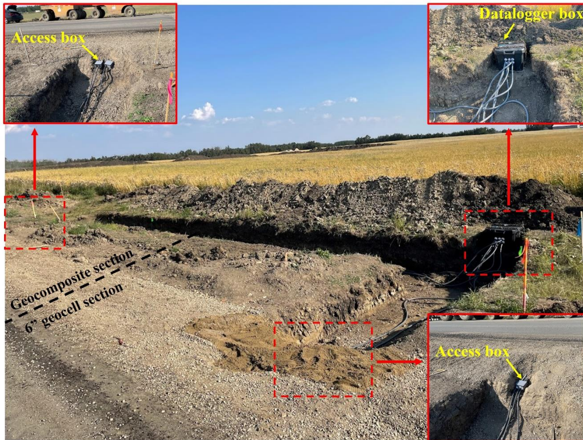
Fig. 5.22. Trench excavation for connecting cables in 6-inch geocell and geocomposite sections
