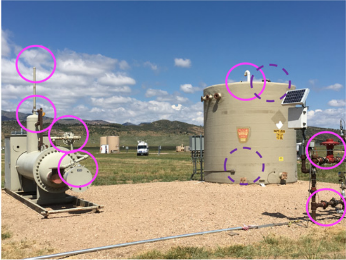
Figure 3.1: Typical methane leak locations in an oil and gas facility
