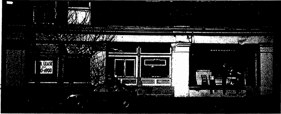
(Photo 47) Detail of the Wilson Building entrances in 1998 pre-renovation.
