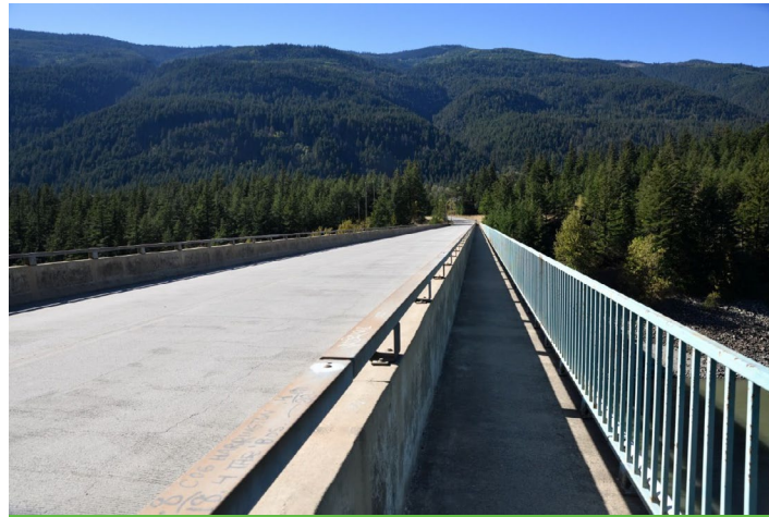
Figure 8: This photo shows the Cog Harrington Bridge that crosses the Fraser between Boston Bar and North Bend. Photo credit: Dr. Francis Zwiers.
