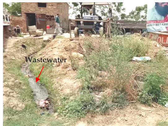
Figure 4. Car Wash Station at Mehat village in India: (a) place of installation of LID system; (b) car washing site.
