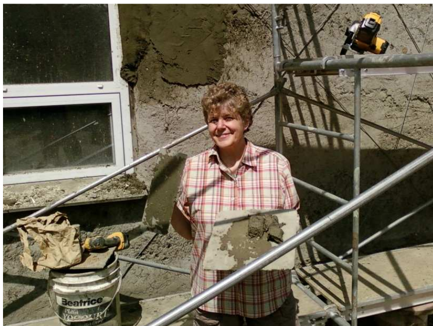
Figure 1: Me Applying Plaster to the Robinson's House
