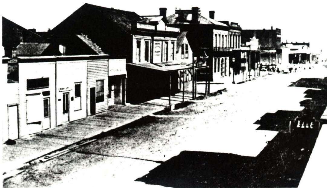
Plate 6. The west side of Government Street, looking north from Fort. The first major building is the Theatre Royal, and next is the Bank of British Columbia, previously the residence of Thomas Harris, the first mayor of the city.
