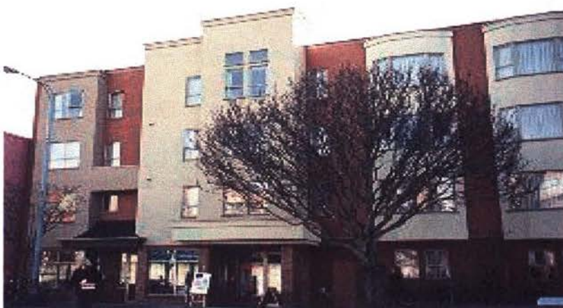
Photo 8: Pandora House Project: A 32 unit supportive housing complex for street people.
