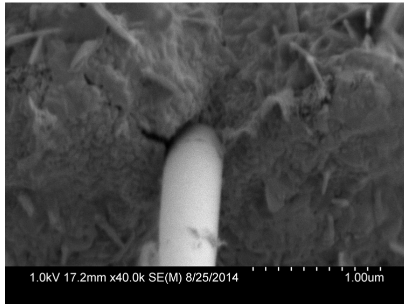
Figure 6.12: A cracked clamp.
