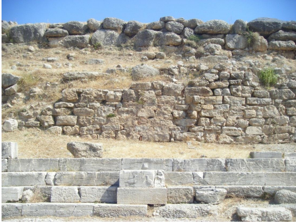
Figure 20 - Detailed view of temple terrace (note difference between eighth century B.C.E. architecture [top] and fifth century B.C.E. [bottom])
