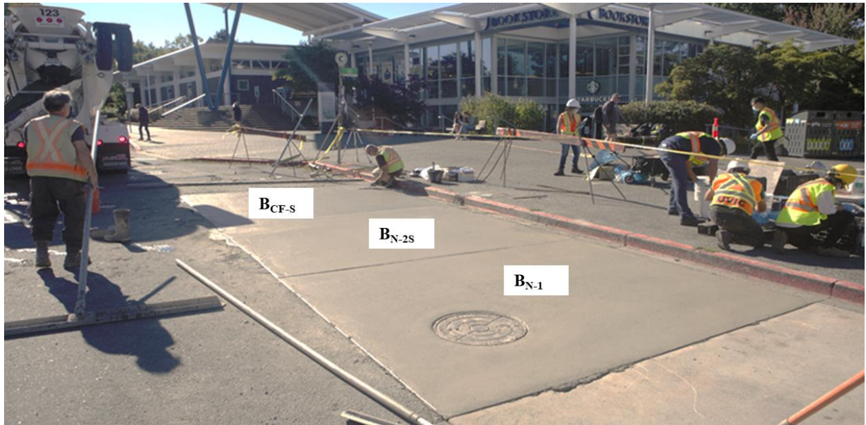
Figure 70. Finished bus pads
