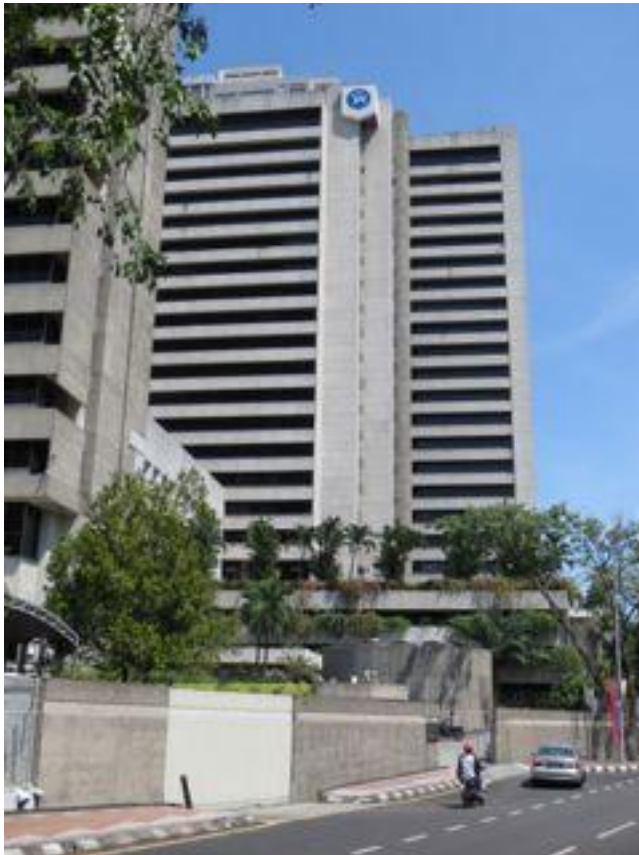
Figure 1: The headquarters of Malaysia’s central bank, Bank Negara Malaysia (BNM).
