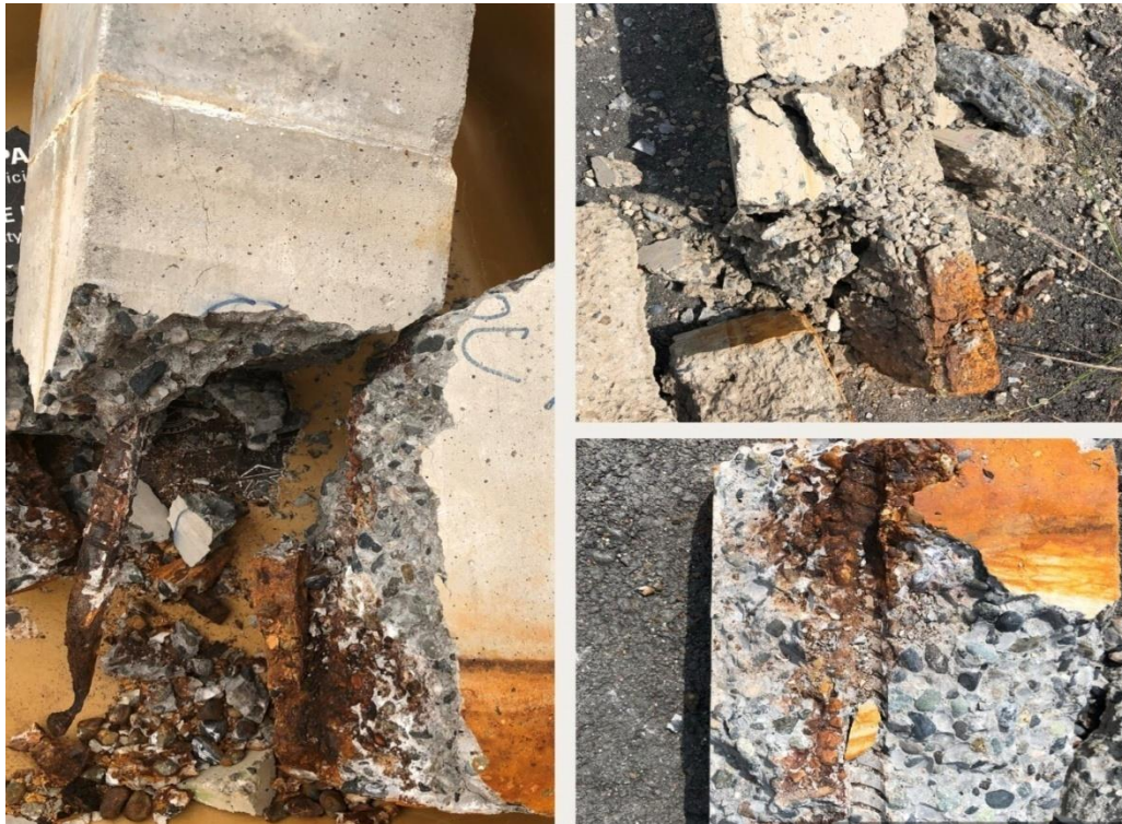
Figure 20 Broken OPC and GPC Beams
