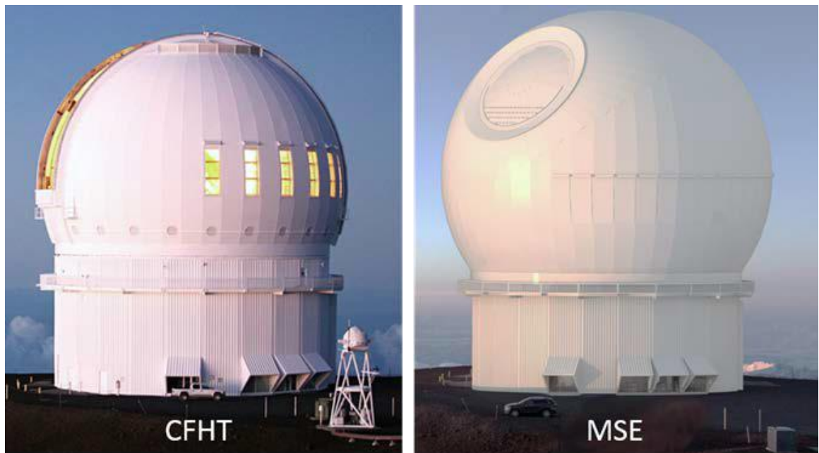
Figure 1.1: Exterior views of CFHT (ventilation modules open) and MSE (ventilation modules closed). Courtesy of Kei Szeto MSE Project Office.
