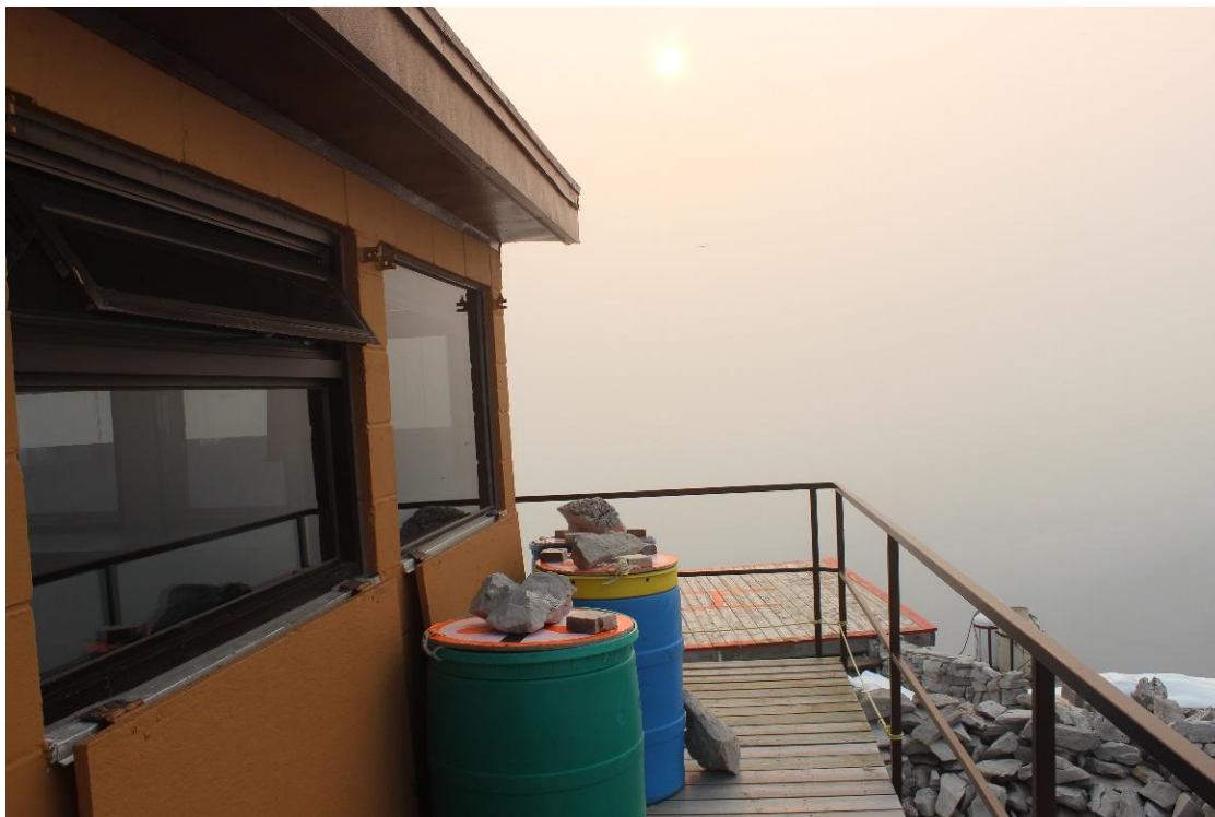
Figure 37. Rain barrels weighted down. This helps to avoid lids and barrels blowing away. (Courtesy: Author).
