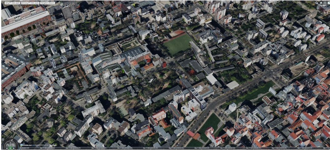
Figure 3.20: The urban scene from a bird's eye view loaded through 3D Web Client/Cesium based on original latitude and longitude points.
