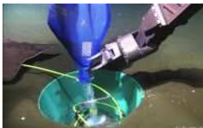
(c) Filling caisson with glass beads.
