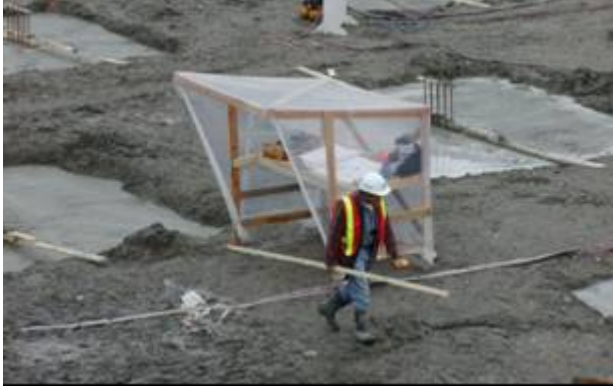
(a) Construction worker and on-site project information.
