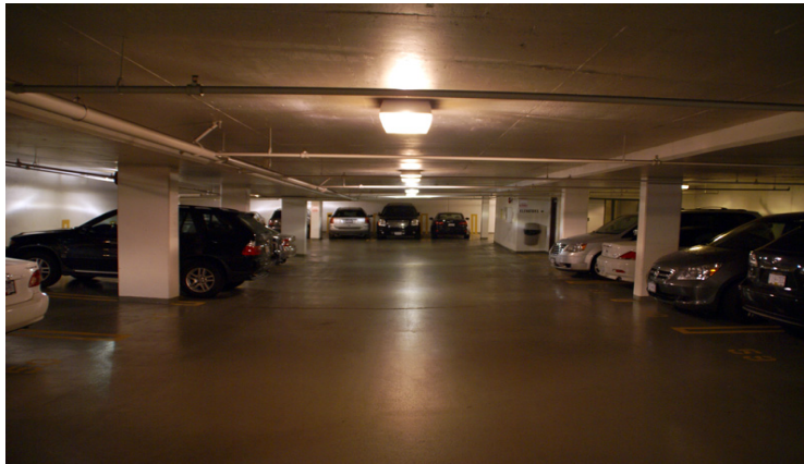
Figure 2.2: A photograph of the multi-level underground parking area used in the demonstration and pilot scale installations of the ILS. A section of the original lighting installation is shown, in total consisting of 89 x 140 Watt MH HID luminaires. The very limited spectral coverage of MH lighting is evident by the orange hue and poor colour rendering of the vehicles in the image, as well as poor contrast between directly lit and shaded areas (these 89 MH HID luminaires were replaced by 52 white LED luminaires at the pilot stage).
