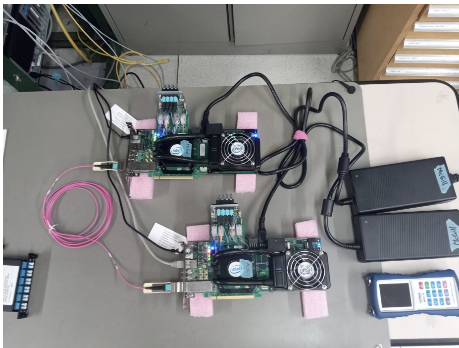
Figure G.3: 2 Intel Stratix 10 FPGA development kits connected together via fiber optic cables. One devkit acts as an Injector of FEB2 data while the other acts as a LASP.
