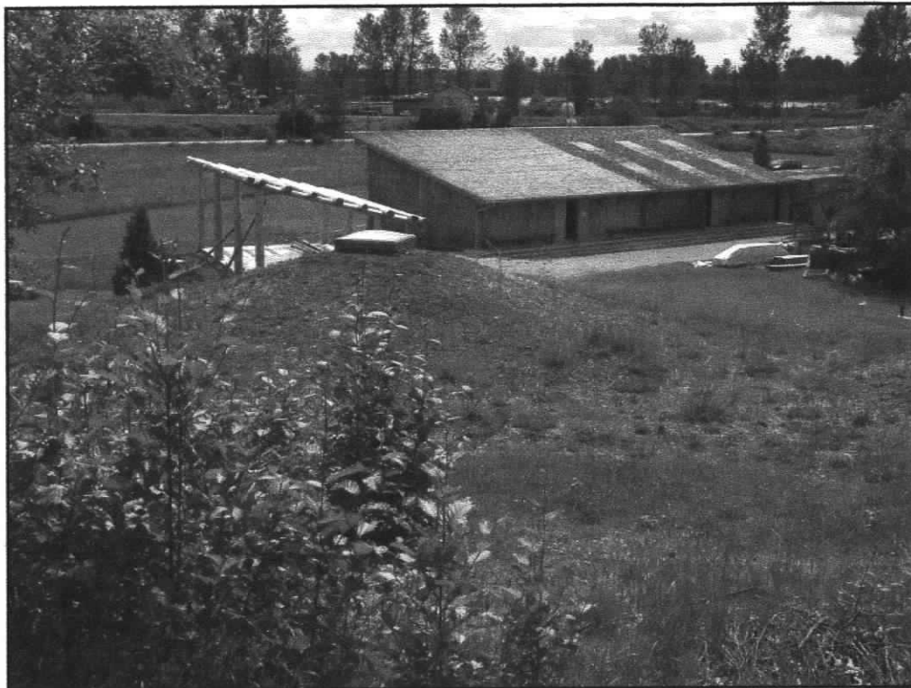
Figure 10: View of the Xa:ytem Longhouse Interpretive Centre (background) and skylight of one of the pithouses (foreground). To the left of the longhouse is another longhouse under construction which will eventually provide an area for canoe carving.
