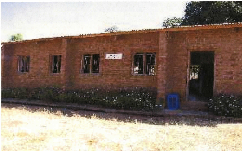
Figure 18. Front view of the main structure for children at the Village-to-Village CBCC Centre showing the size and type of construction materials used.
