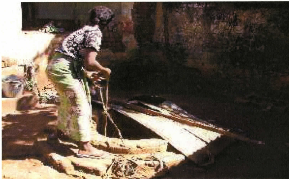
Figure 14. The deep well at Namikango CBCC Centre, the proximity of the well to the main building and the tattered iron sheet used to cover the mouth of the well.
