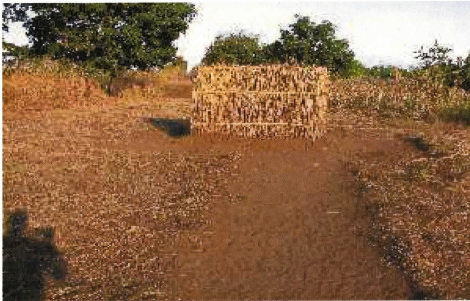
Figure 12. From a distance, an enclosed pit latrine used by both the caregivers and the 150 registered children of the Lomoni CBCC Centre.
