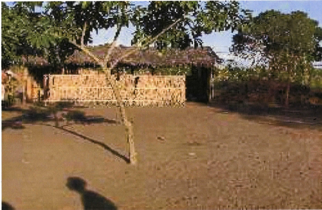
Figure 2. Distant view of the main structure of Lomoni CBCC Centre depicting the construction materials and the size.
