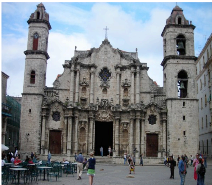
2.1 The Havana Cathedral (1748-1777), view from the back of the plaza.
