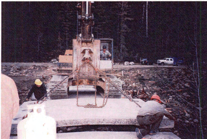
Figure 4.20 - Precast Panel Erection
