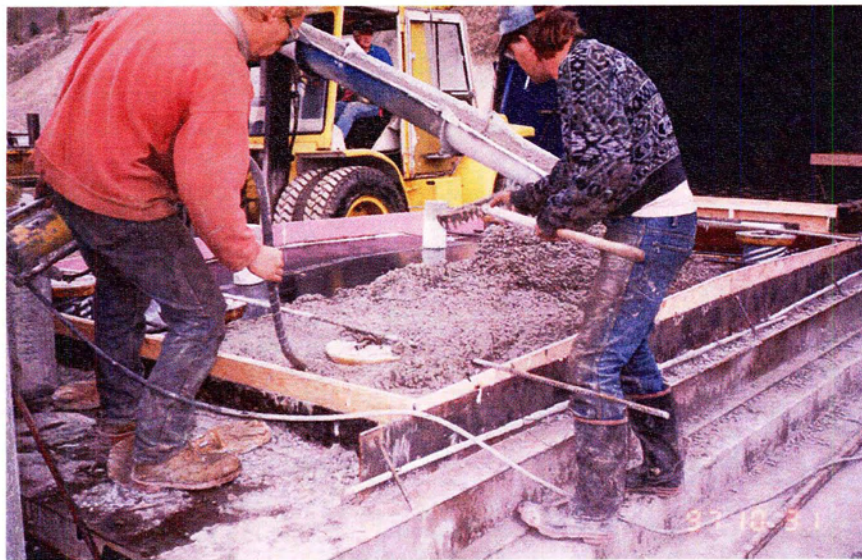
Figure 4.19 - Precast Arch Panel Fabrication
