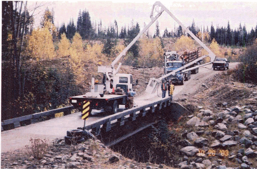
Figure 4.35 - Bridge Inspection Vehicle. A Logging Truck Typical of the Road use can be seen on the East Approach to the Bridge
