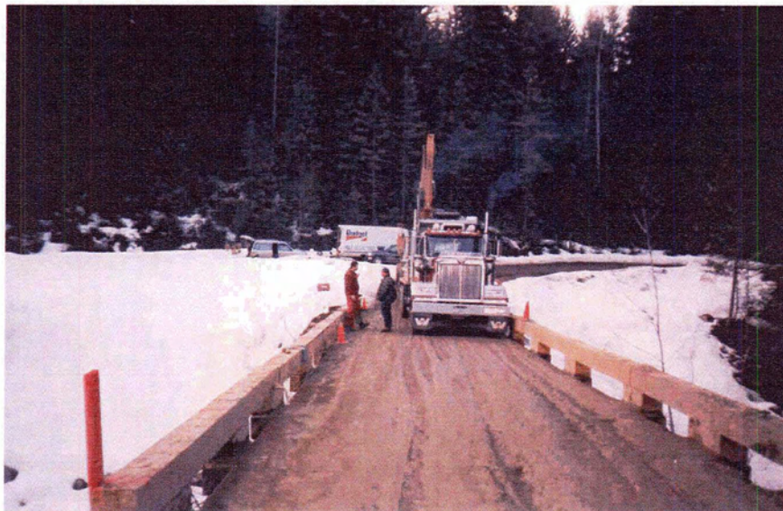
Figure 4.29 - Test Vehicle in Left Position (Monitoring Station in Background)
