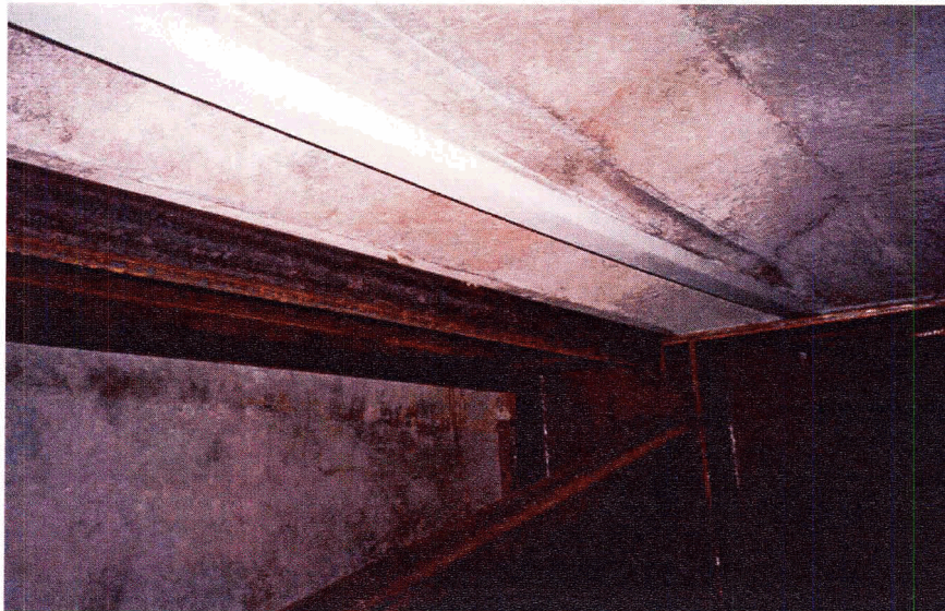
Figure 4.23 - Underside of Deck showing Steel Channel for Transverse Edge Stiffening
