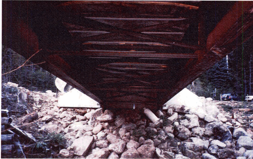
Figure 4.22 - Underside of Deck showing Steel Straps
