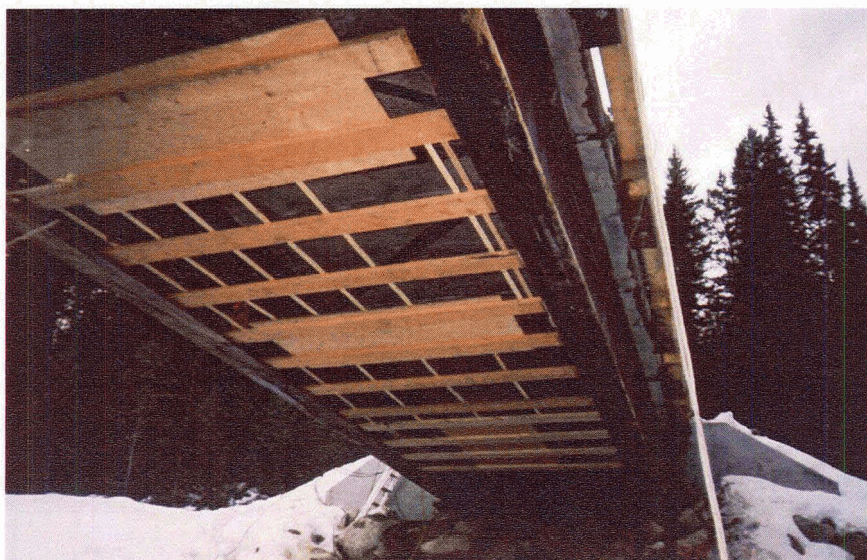
Figure 4.30 - Access Platform beneath Deck
