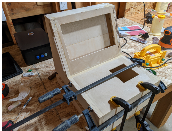
(b) Adding facades to the kiosk.
