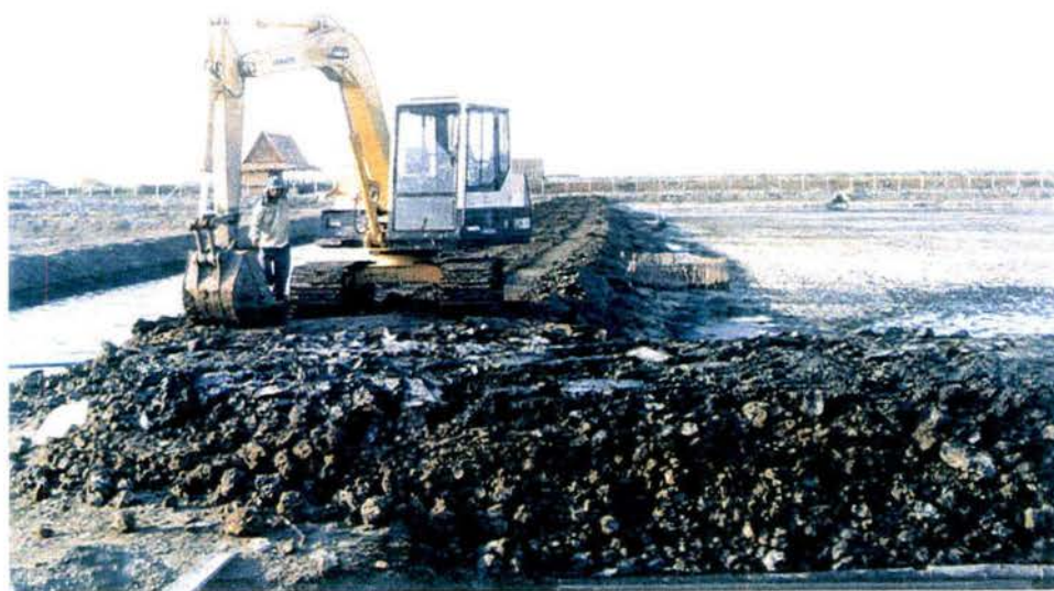
FIGURE 19. HEAVY MACHINERY COMMONLY USED TO REPAIR OR MODIFY SHRIMP PONDS, REMOVE ACCUMULATED SEDIMENT AFTER DRY-OUT AND CONSTRUCT DRAINAGE CANALS
