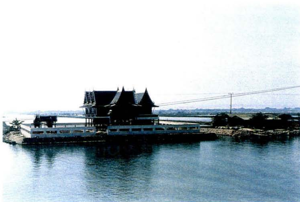
FIGURE 24. PITTHAYALONGKORN CANAL AND EXTENSIVE SHRIMP POND IN THE BACKGROUND. THE HOUSE IS OCCUPIED BY A PREVIOUS SAMUT SAKHON INTENSIVE SHRIMP FARMER
