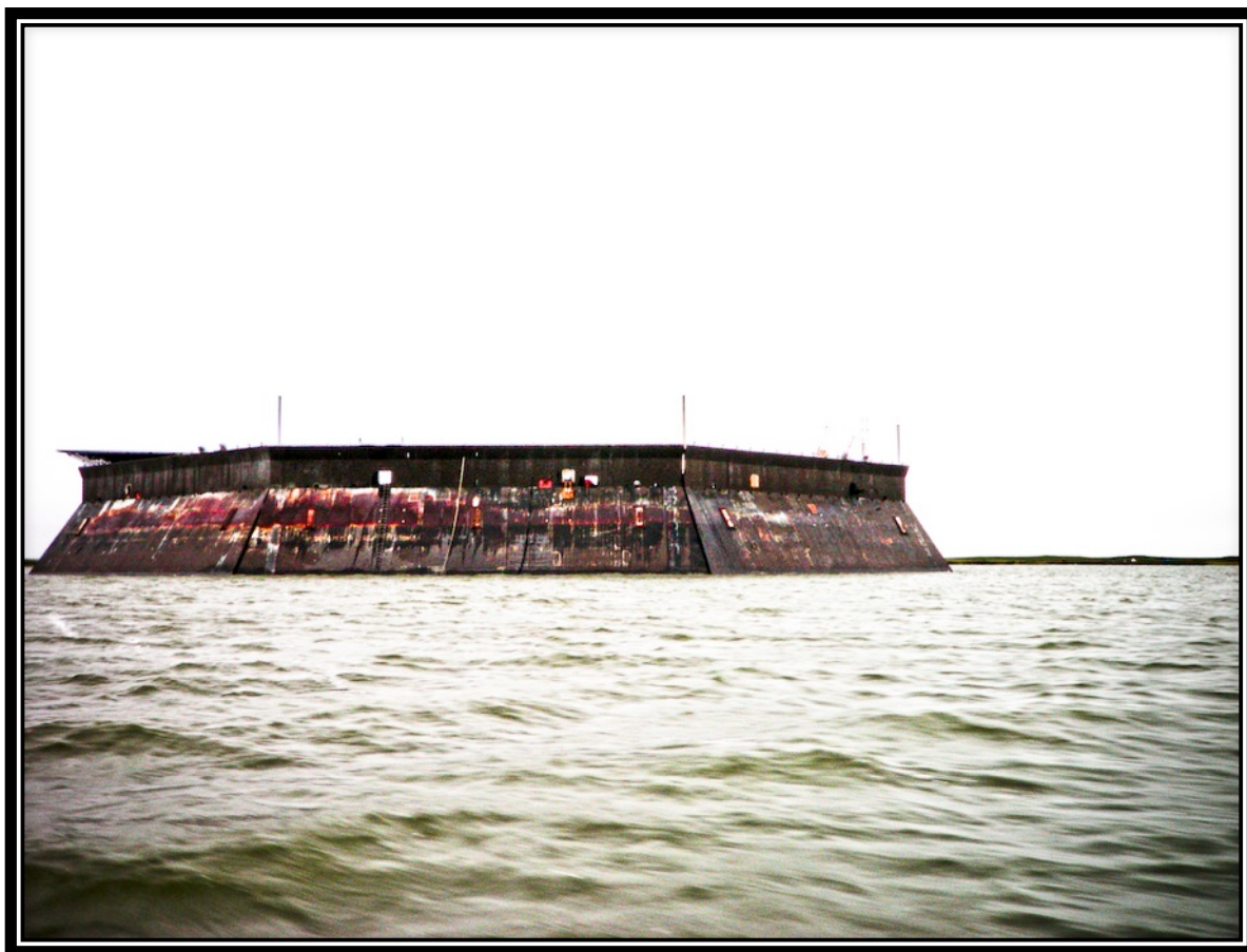
Figure 1.5 A photo of a protective platform once used to protect oil exploration/drilling activities from winter sea ice in the Beaufort Sea, is now abandoned in Tuktoyaktuk harbour. Near Tuktoyaktuk, NWT. Photo by T.D. Bennett, 2010.
