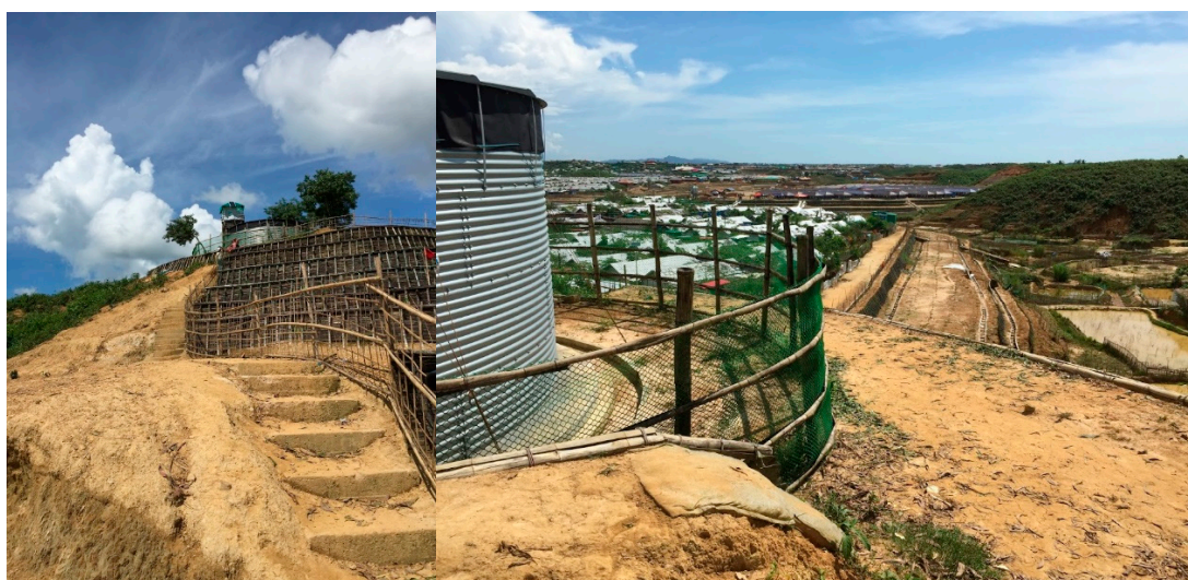
Figure 2. Water supply tank in Camp 4Ext, October 2019, Credit: SMN Uddin.
