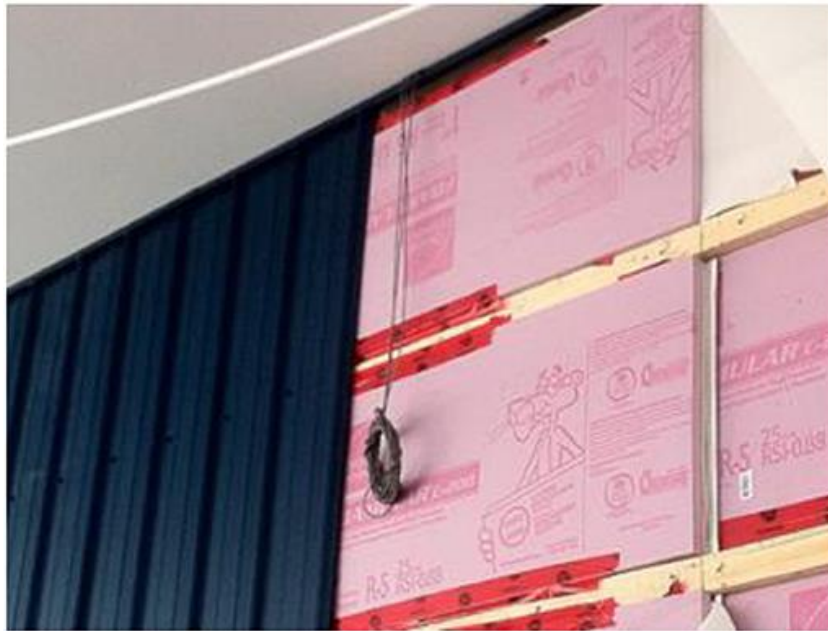
Figure 5. The second layer of XPS is shown in place over 6 mm polyurethane foam. The XPS layer ensured that the bottom surface of each VIP was attached to a smooth surface and protected from abrasion. A layer of 6 mm flexible polyurethane foam was placed over the exterior surface of the VIPs to help prevent mechanical rubbing of the outside surface of each VIP against the 25 mm polystyrene foam board placed on top of it.
