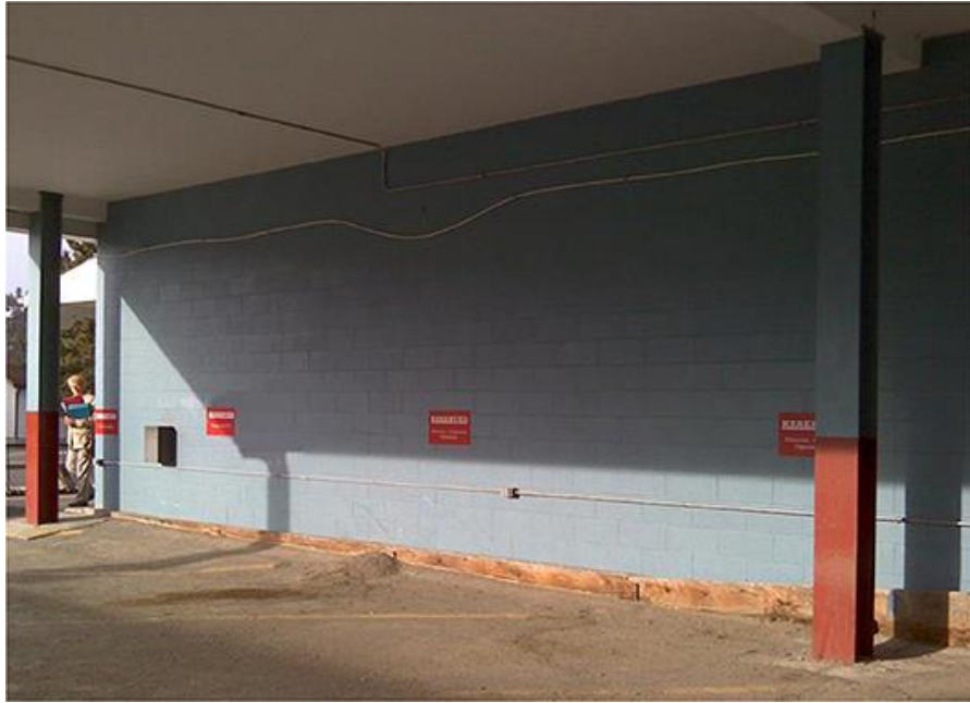
Figure 3. Existing wall selected for retrofit [11].
