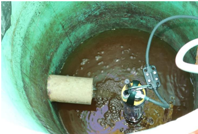
Photo 5. Effluent draining into sediment trap and YSI deployed
