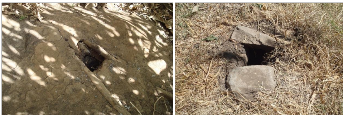
Figure 26 - Conventional Dry Latrines with no Cover / Lid
