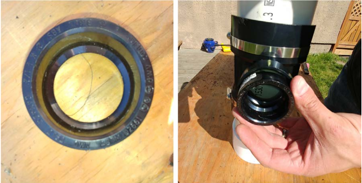
Figure A.29: Installation of the bushing on the tee fitting.
