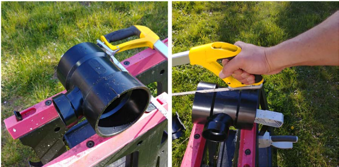
Figure A.28: Cutting of the tee fitting.
