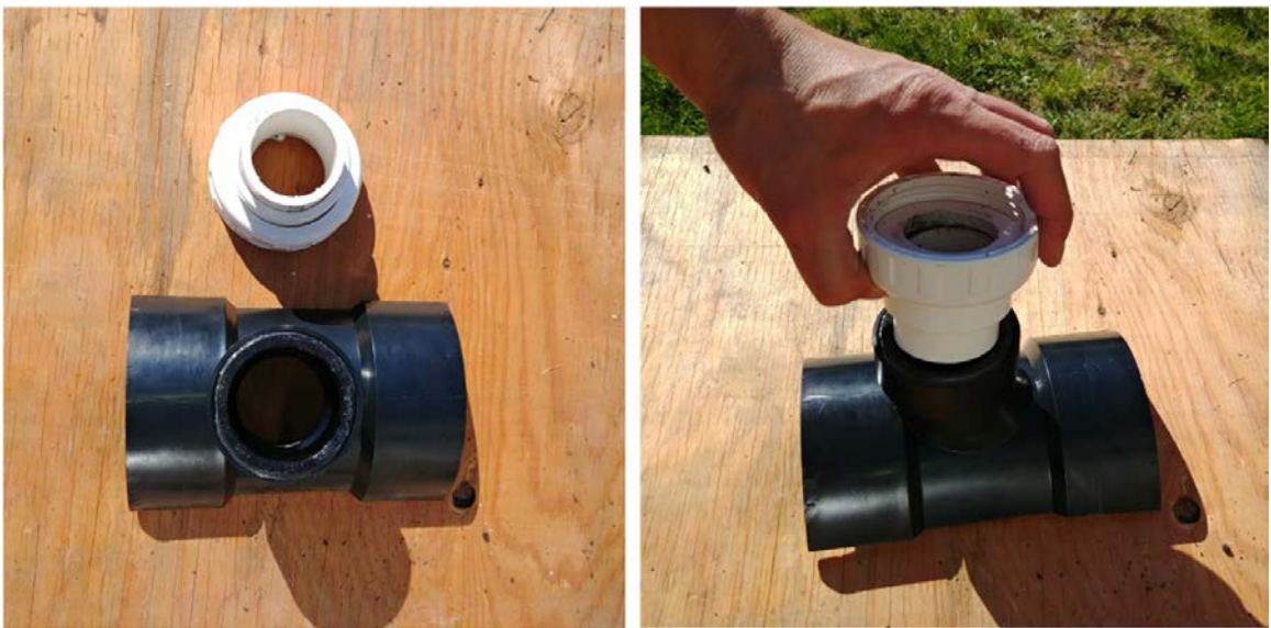
Figure A.30: Installation of the PVC union fittings.
