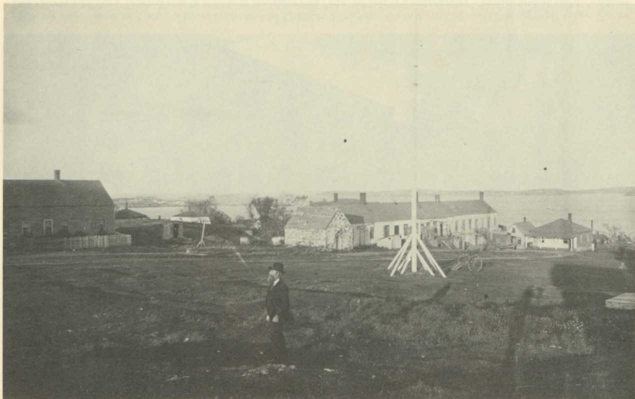
Looking northeast from Commander's House at Fort Sullivan, with former Powder Magazine, Soldiers' Barracks, and Hospital at center. Photograph taken during 1900 survey of Fort. (From the National Archives).
