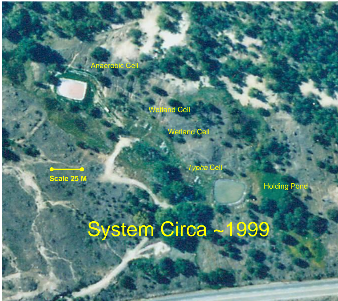
Figure 3. Aerial photograph of wetlands in 1999 showing the 5 treatment cells (Note: anaerobic cell pink due to rhodamine dye test for HRT determination).
