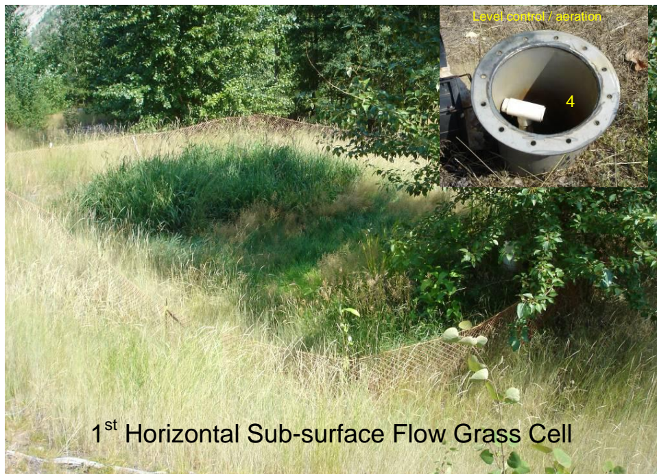
Figure 7. First wetland cell in summer 2009 showing aeration chamber and sampling point.
