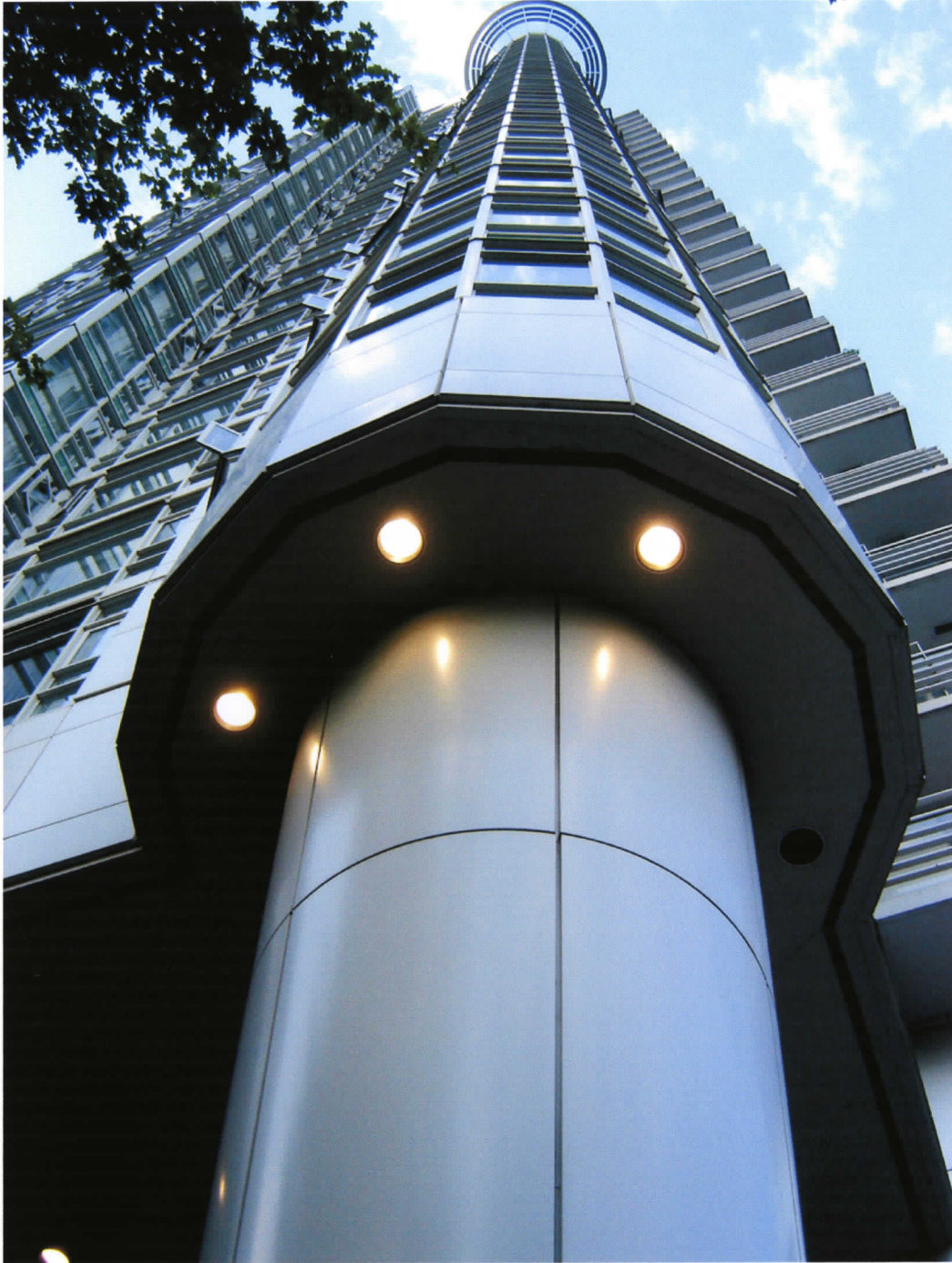
Fig. 26. James K.M. Cheng Architects Inc., Aquarius II on the northeast corner of the Aquarius project, Vancouver, 1999. View from the northeast (Photo: Menno Hubregtse).
