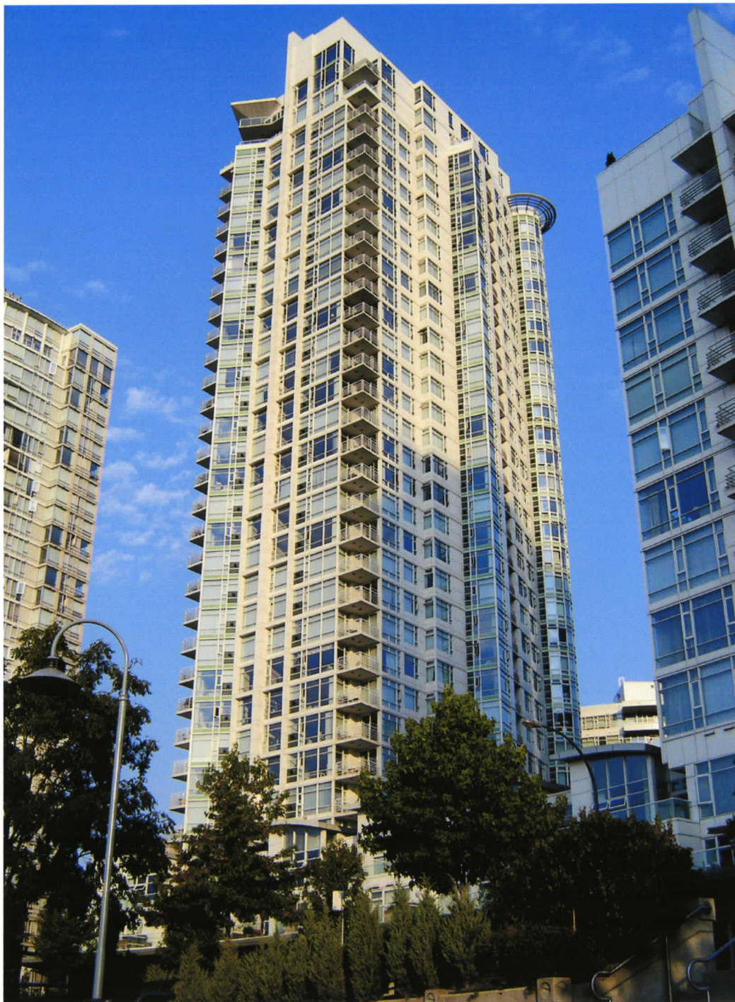
Fig. 30. James K.M. Cheng Architects Inc., Aquarius I on the south-southwest corner of the Aquarius project, Vancouver, 1999. View from the east-southeast (Photo: Menno Hubregtse).
