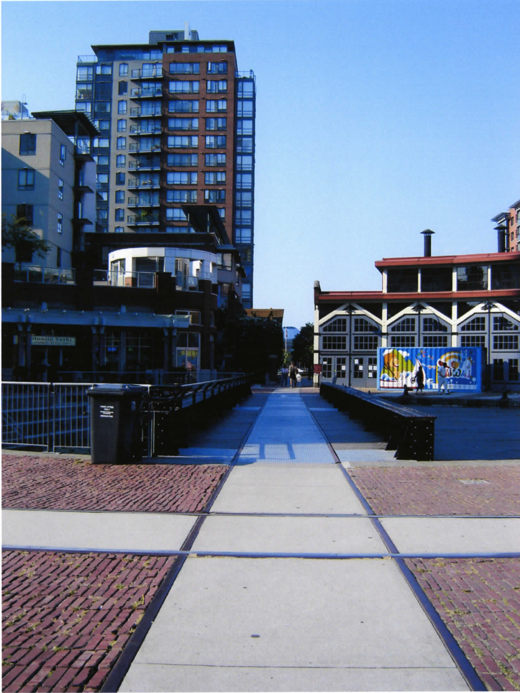
Fig. 10. CPR Engine Turntable, Vancouver, 1889. View from the northeast (Photo: Menno Hubregtse).
